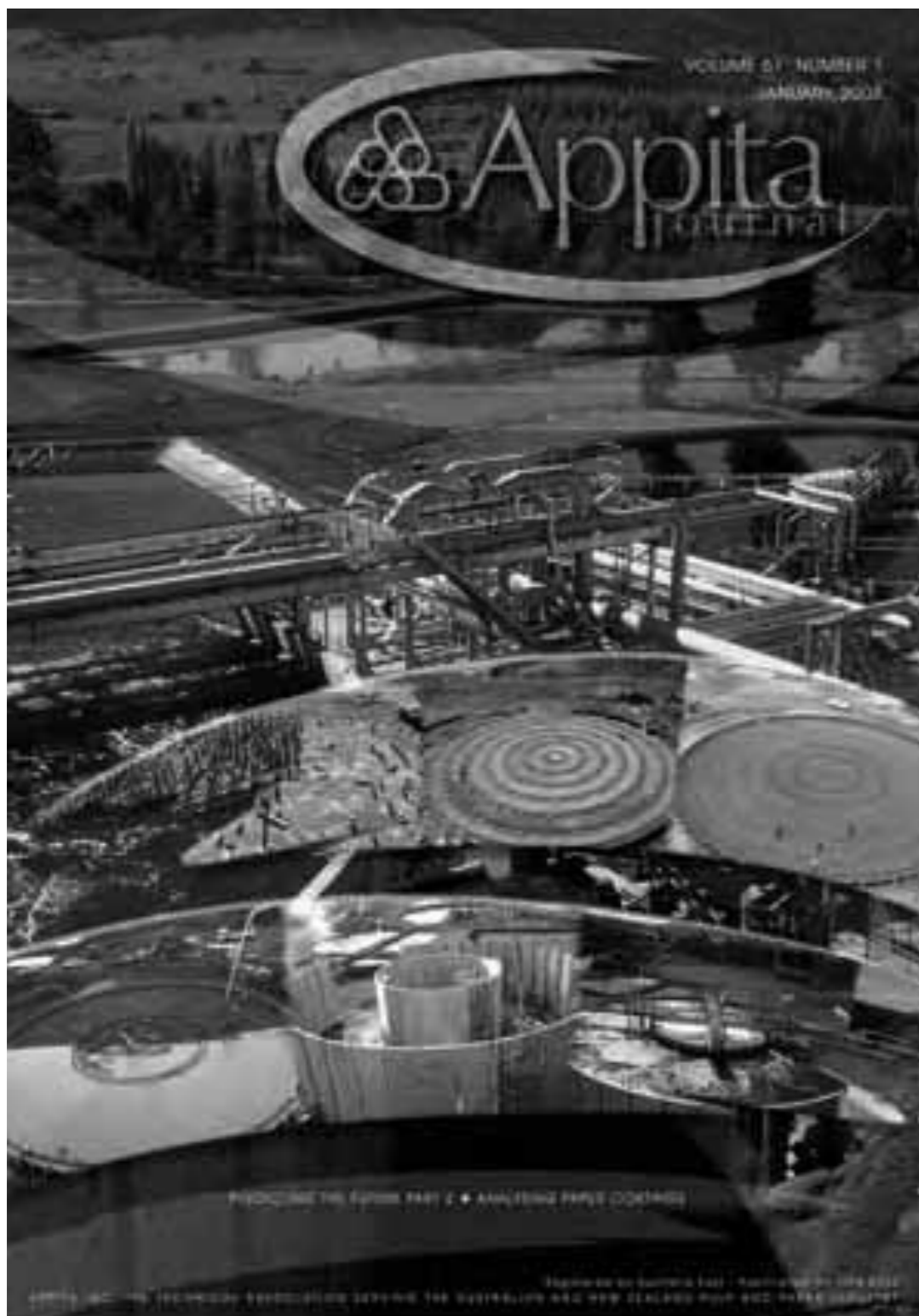
Cover: Norske Skog Boyer's Secondary effluent treatment plant. Photographs courtesy Norske Skog Boyer. See feature on page 6.
