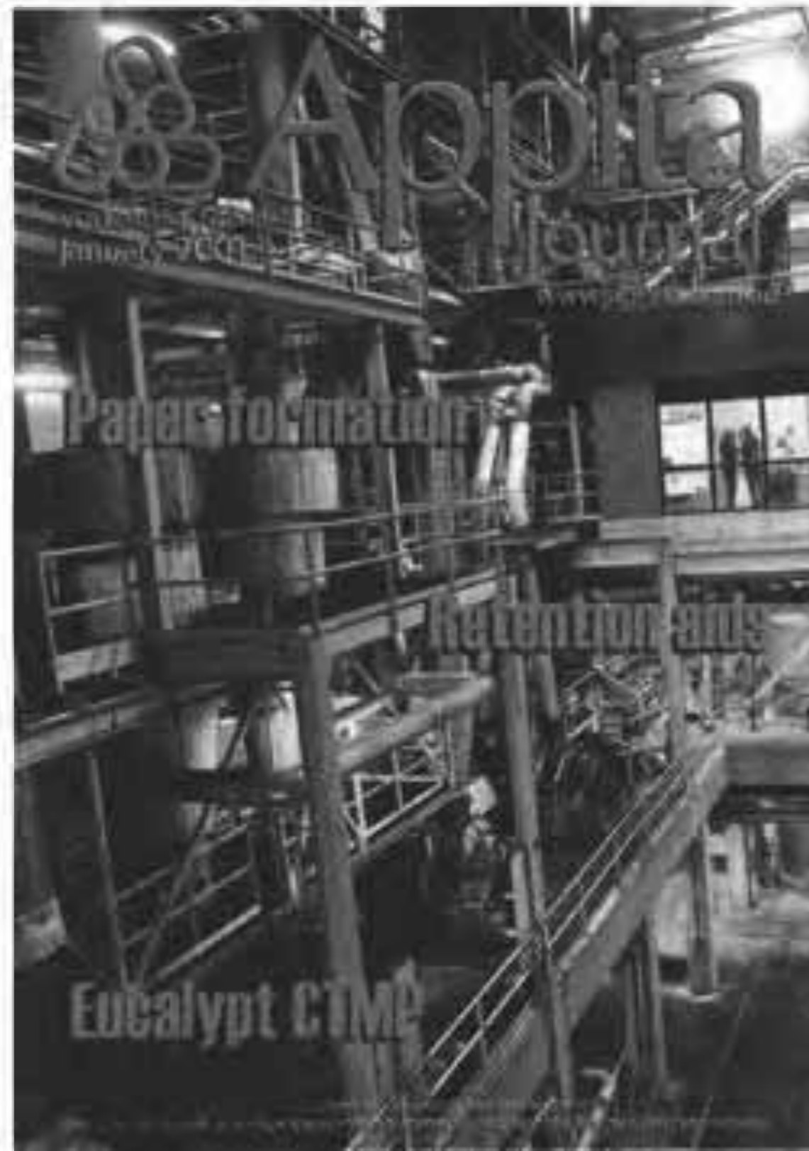
Cover: Norske Skog Albury TMP plant, courtesy Norske Skog. Photograph © Peter Whyte/Creative Partners, 2001.
